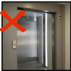
Inaccessible Lift (No Grab bars)
