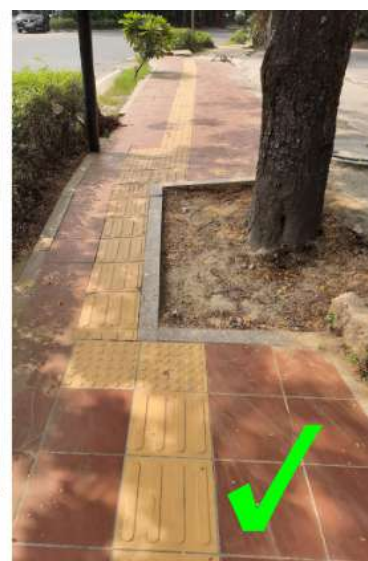
Accessible & appropriate way of laying of TGS
