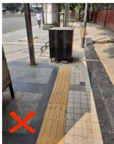
Inaccessible & Improper way of laying of TGS
