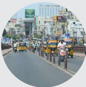
1. Rail Over Bridge near Shankarvilas Centre
