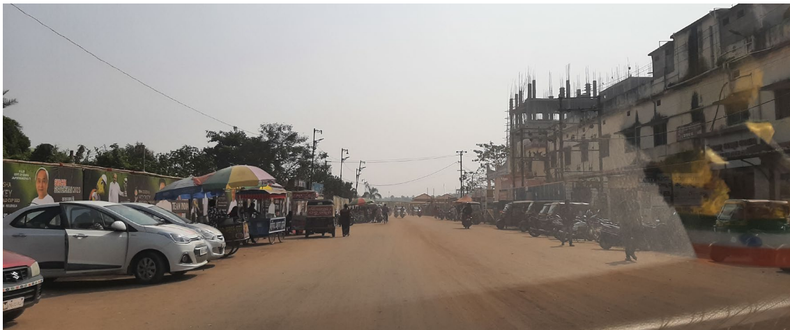
Figure 5: Overhead Electrical Wiring along Kusuma Road Source: UN-Habitat
