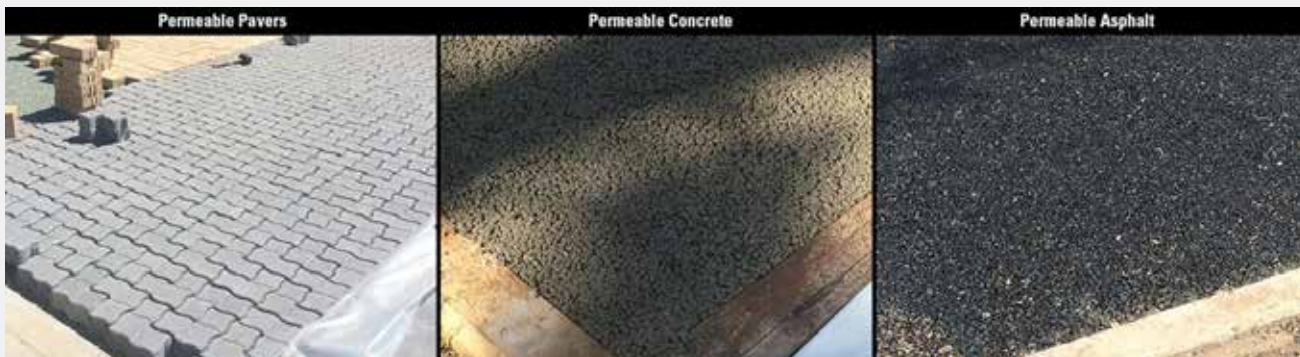
FIGURE 3.59 Types of permeable pavements
