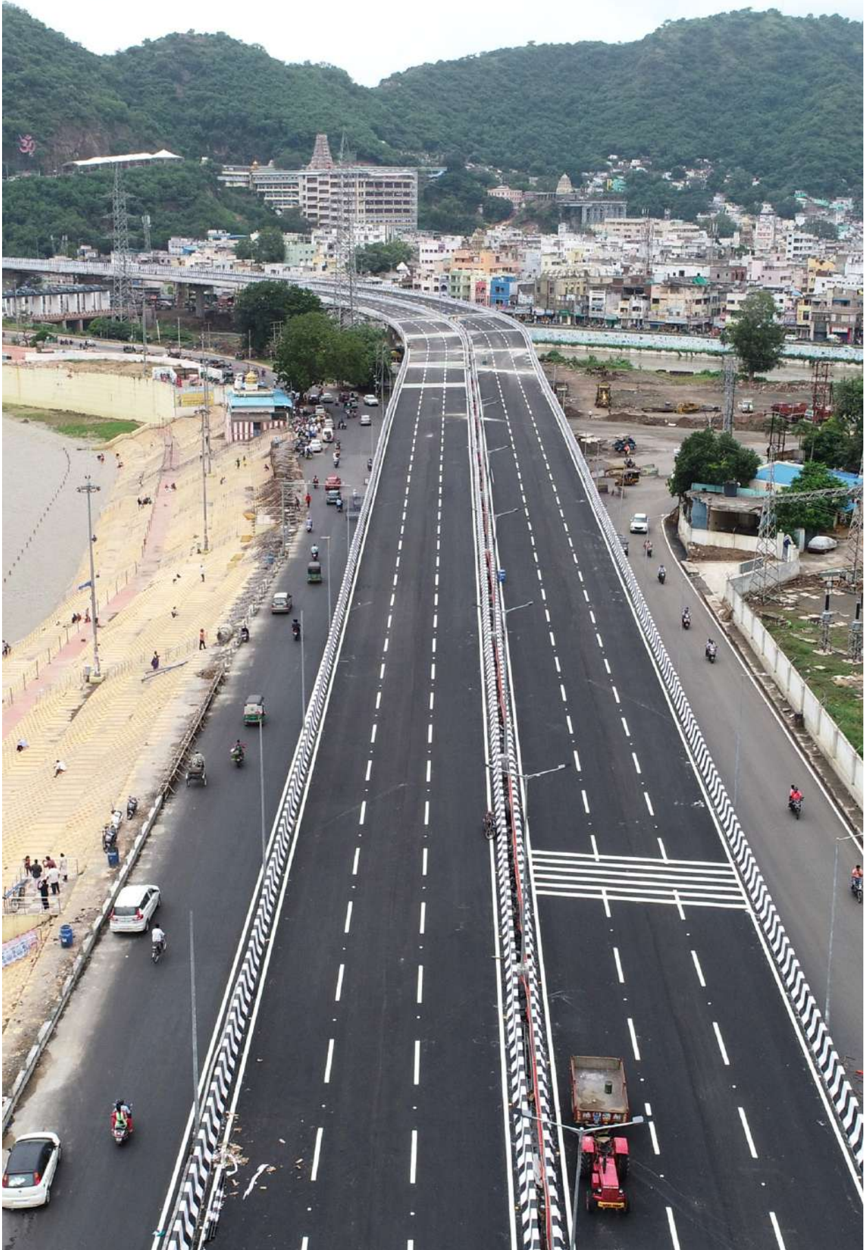
Image 4.22: View of NH-65 and Kanaka Durga Temple flyover near VMC Office
