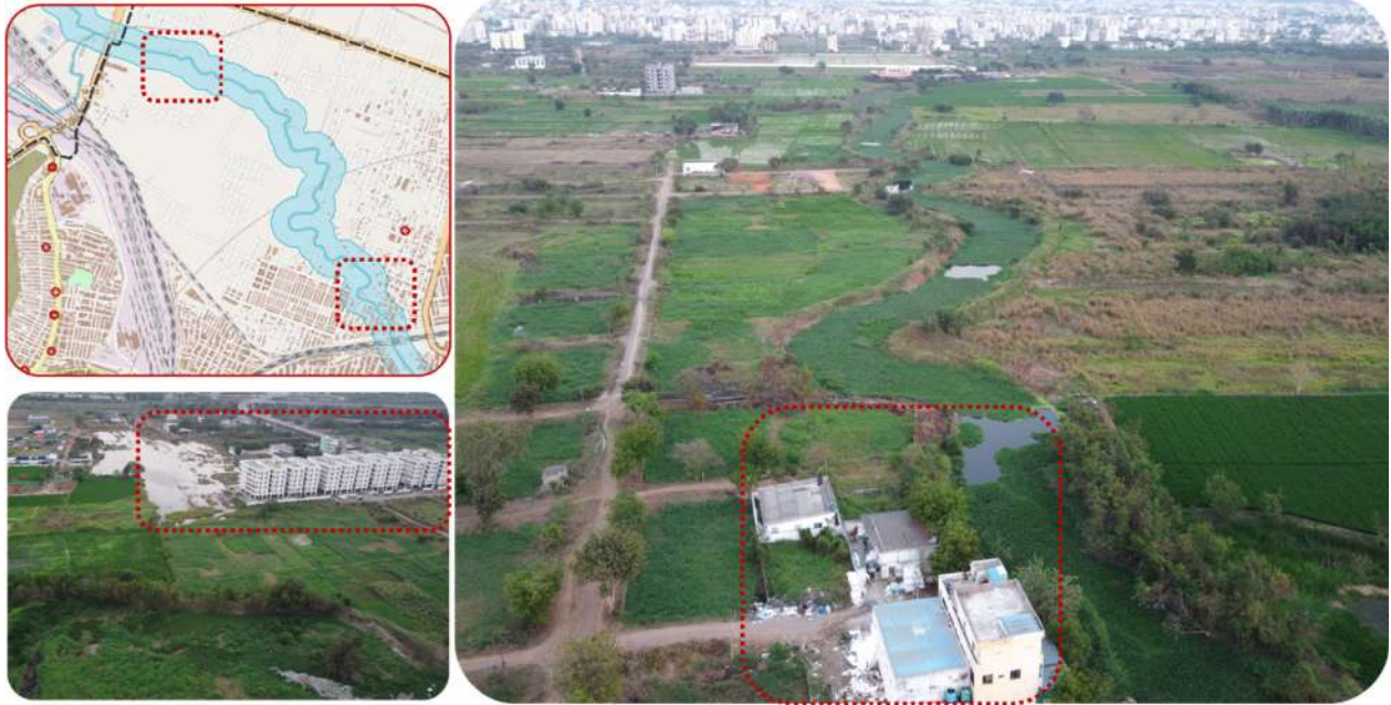
Image 5.7: Unauthorized constructions along Budameru canal to the North-West of the city.
