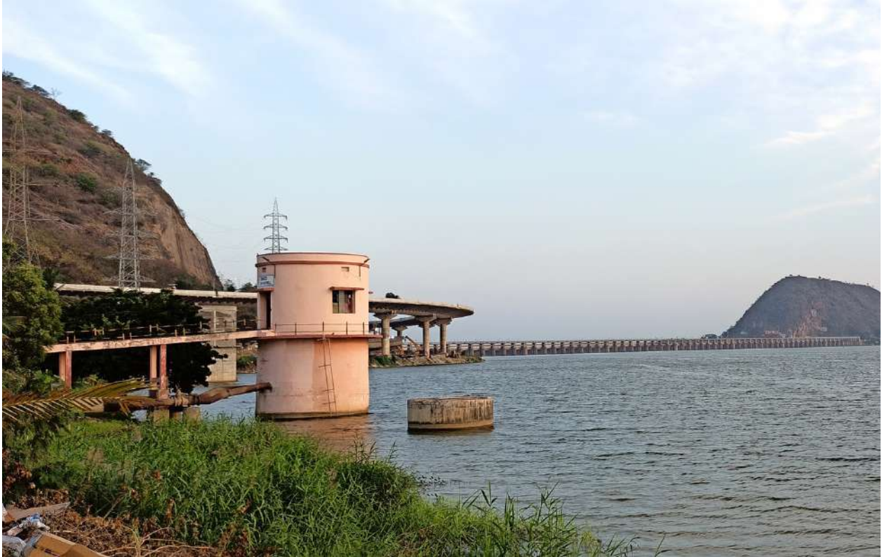
Image 4.16: Head Water Works intake well and treatment plant in Krishna River
