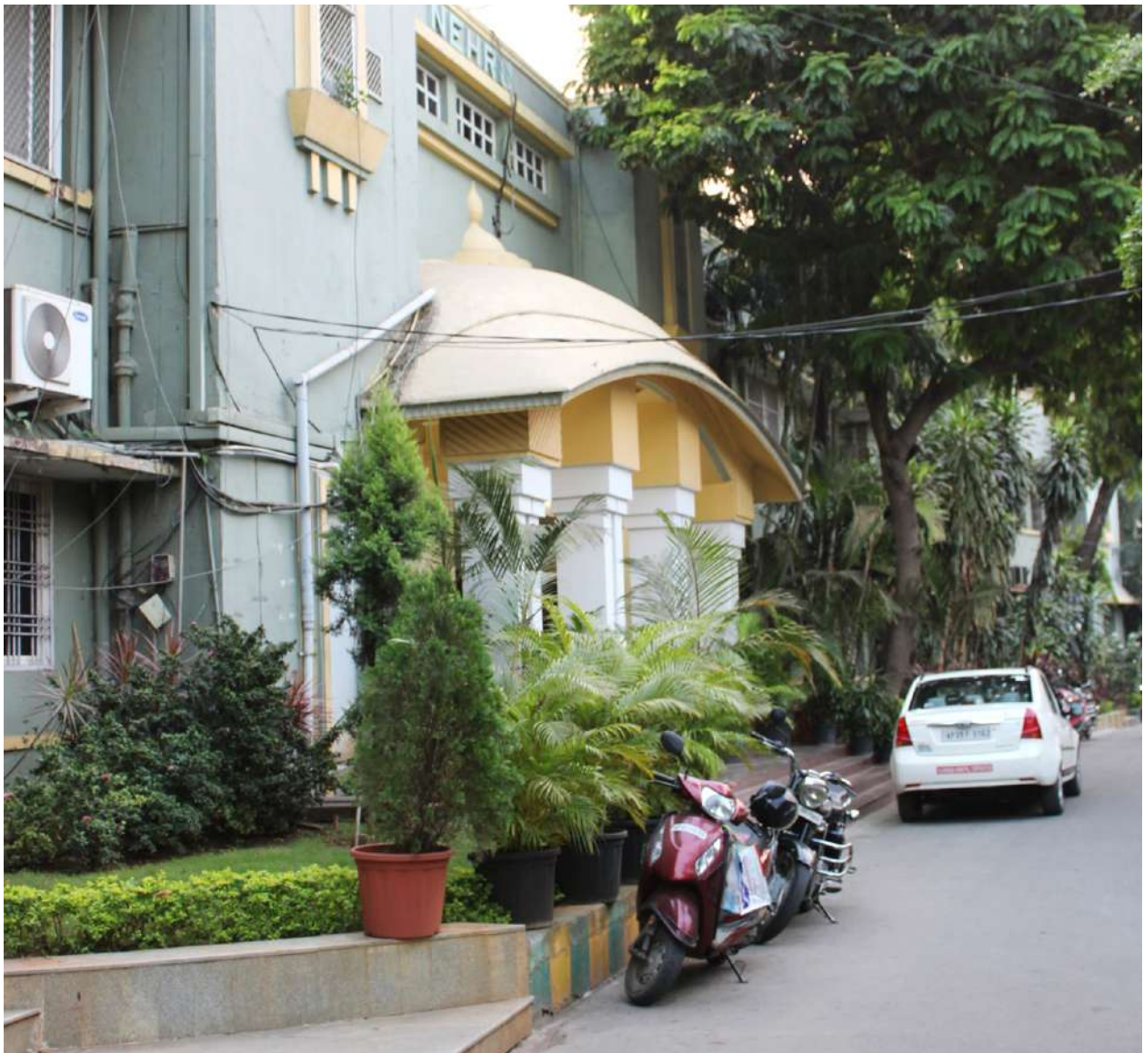
Image 3.1: View of Vijayawada Municipal Corporation office building
