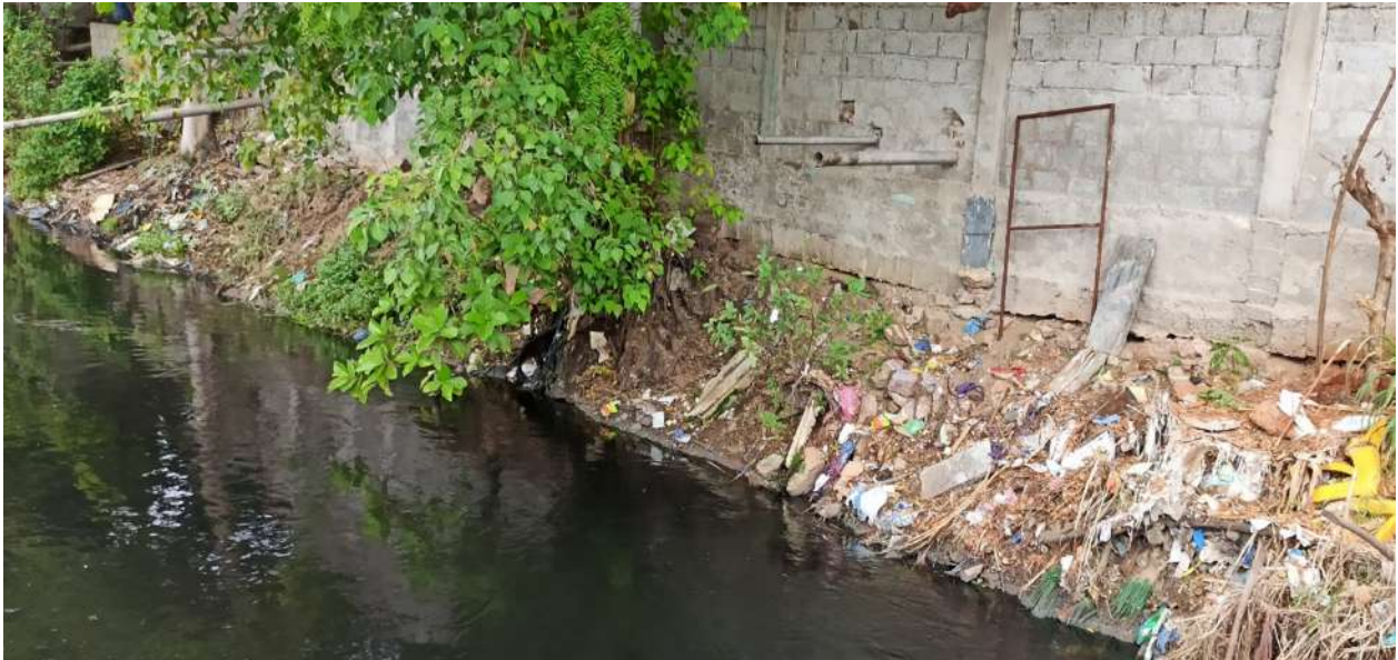
Image 4.26: View of Budameru canal with drainage outlet pipes and solid waste dump
