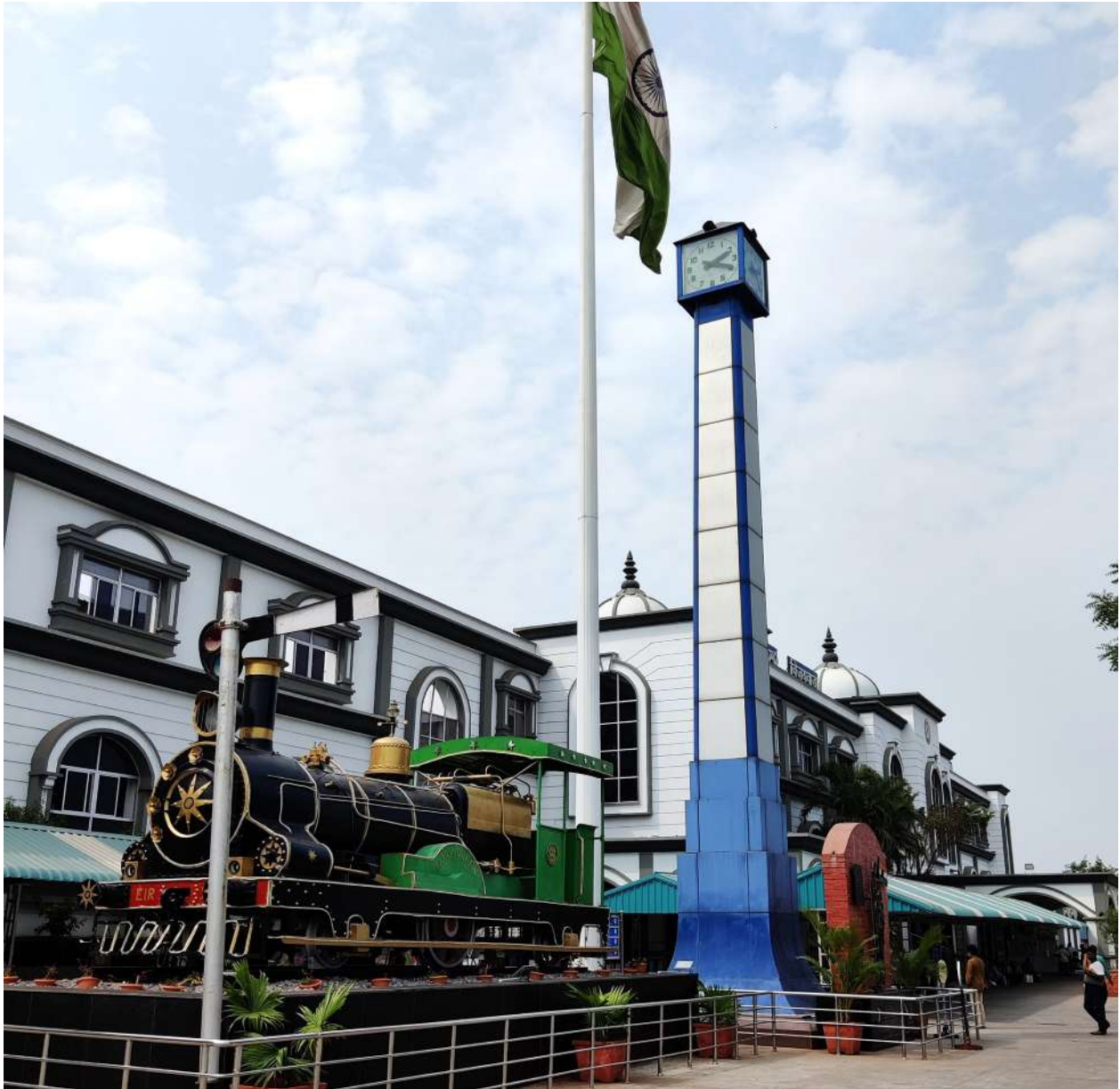
Image 2.1: View of the Vijayawada railway station façade
