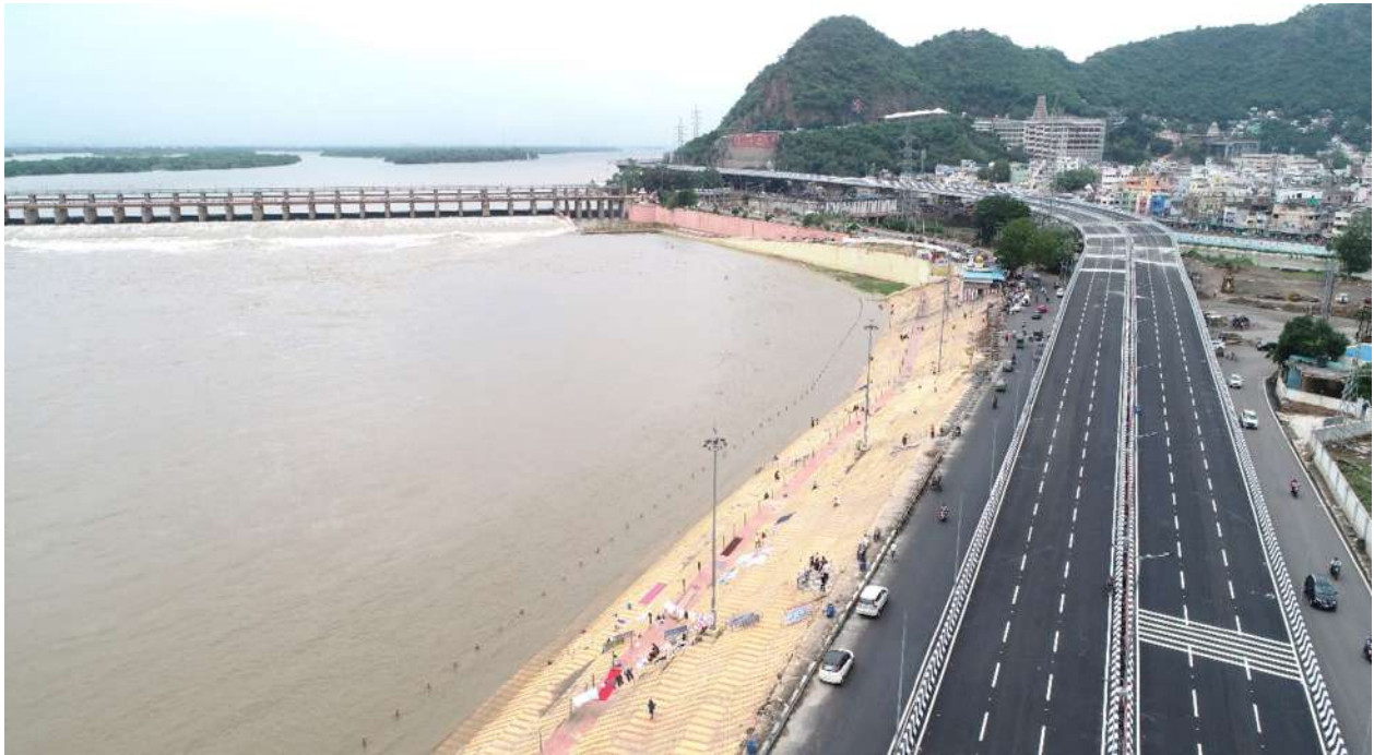
Image 4.1: View of Prakasam Barrage, Indrakeeladri Hill and river ghat for religious activities
