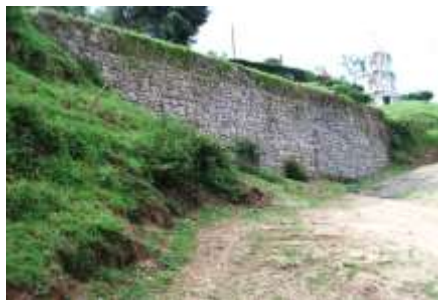
Rock Filled Gabions
