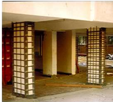
Retrofitting technique of column
