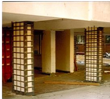
Retrofitting technique of column
