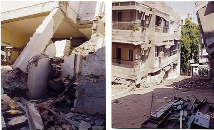
Failure and collapse pattern
