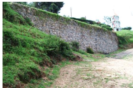
Rock Filled Gabions
