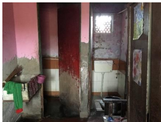
Figure 41: Dwelling unit at Bawana housing, Delhi
