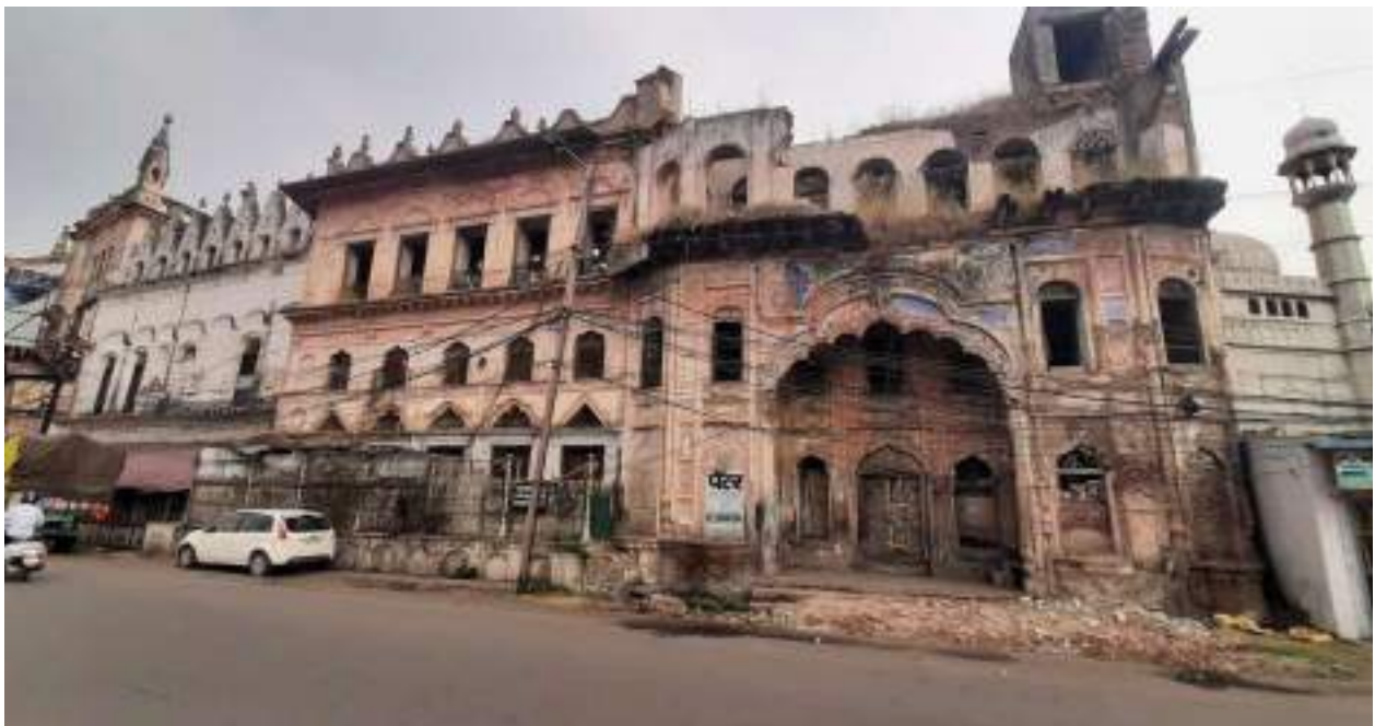
Image 4.3: Shaukat Mahal, a dilapidated heritage structure in the old city
