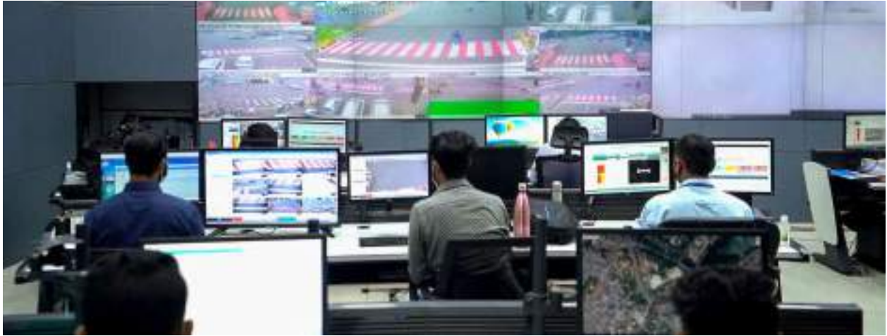
Image 4.17: Control and Command Centre (IOCC) set up under the Smart City Mission at BSCDCL Office in Govindpura
