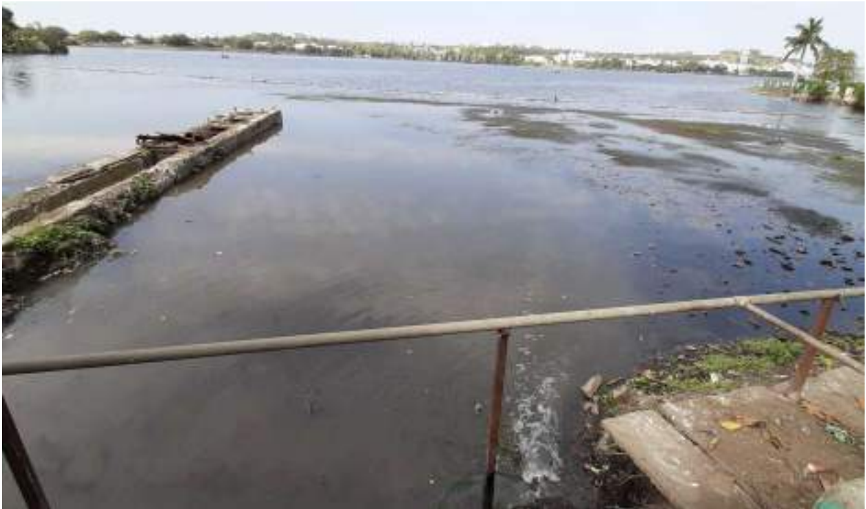
Image 4.8: Sewage inlet to Shahpura Lake for retention and oxidation
