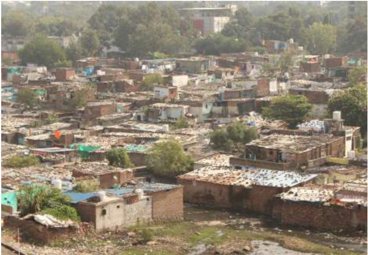
Image 4.6: Banganga Slum Settlement lies in the valley between Upper Lake and Lower Lake
