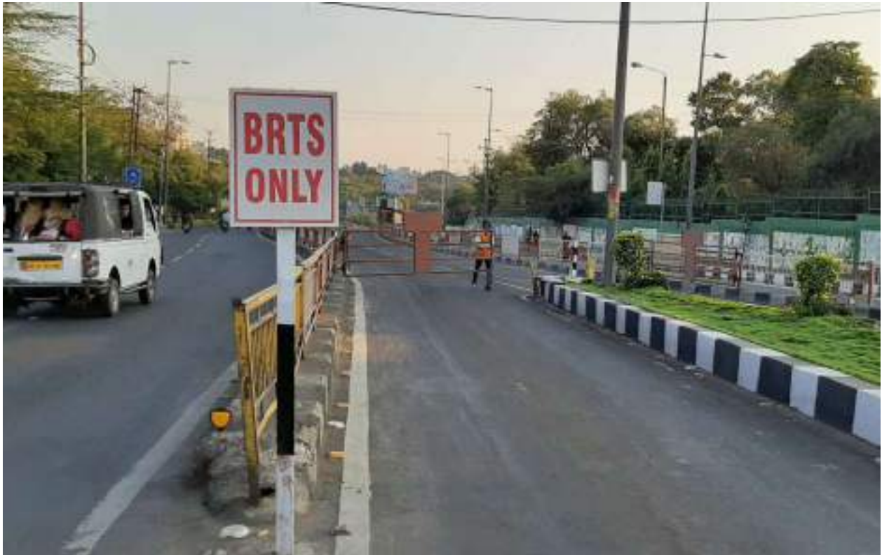
Image 4.12: BRTS corridor near Ravindra Bhavan. The gates are manually operated to prevent entry of other vehicles
