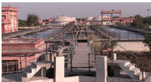
Image 4.15: 62.5 x 2 MLD STP at Delawas
