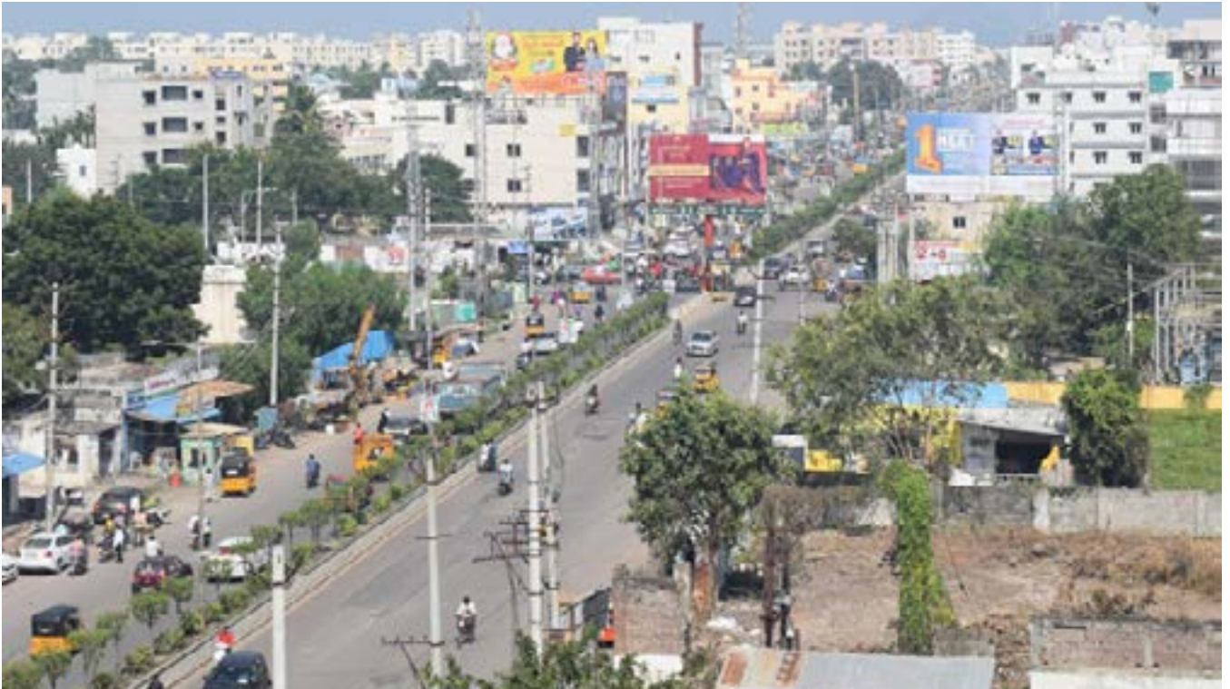
View of Amaravati Road–MG Inner Ring Road Intersection (proposed UGN 1)
